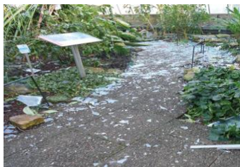
Storm damage has resulted in multiple broken panes of glass in the glasshouses at Inverleith in Edinburgh, leaving tender plants exposed to the elements.
